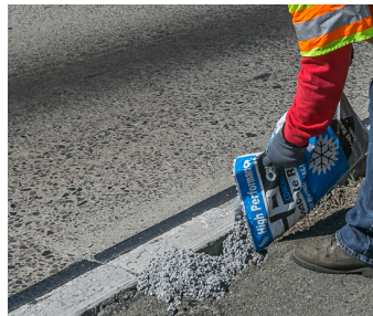
Fill Repair Area
