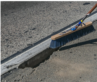
Clean Repair Area
