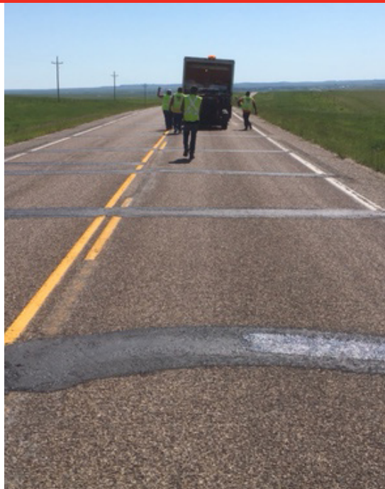
Leveling Depressed Thermal Cracks
