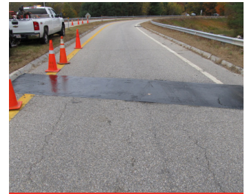
SEALING UTILITY CUTS
