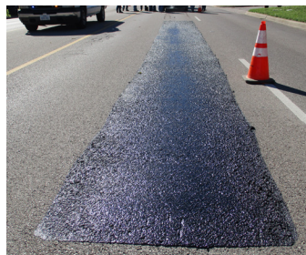
SKIN PATCH REPAIRS
