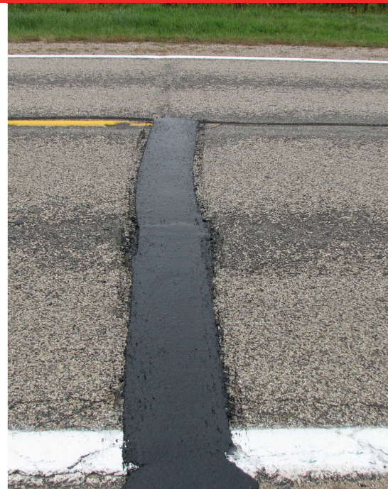
Filling Wide Cracks and Joints
