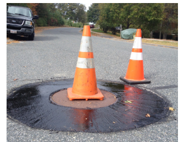
LEVELING MANHOLE COVERS
