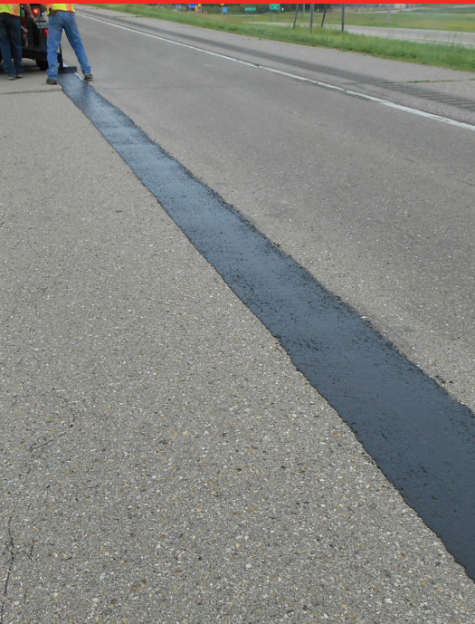
Repairing Deteriorated Longitudinal Joints
