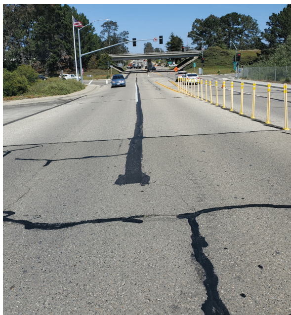
Mastic One cools quickly after installation and is ready for traffic when it has solidified sufficiently to support loads.
