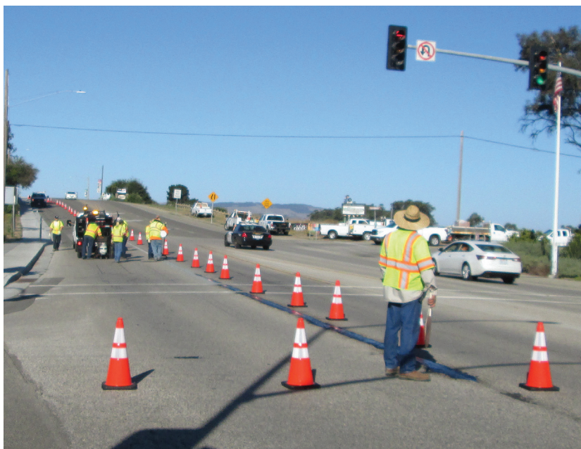
Mastic One cools quickly after installation and is ready for traffic when it has solidified sufficiently to support loads.
