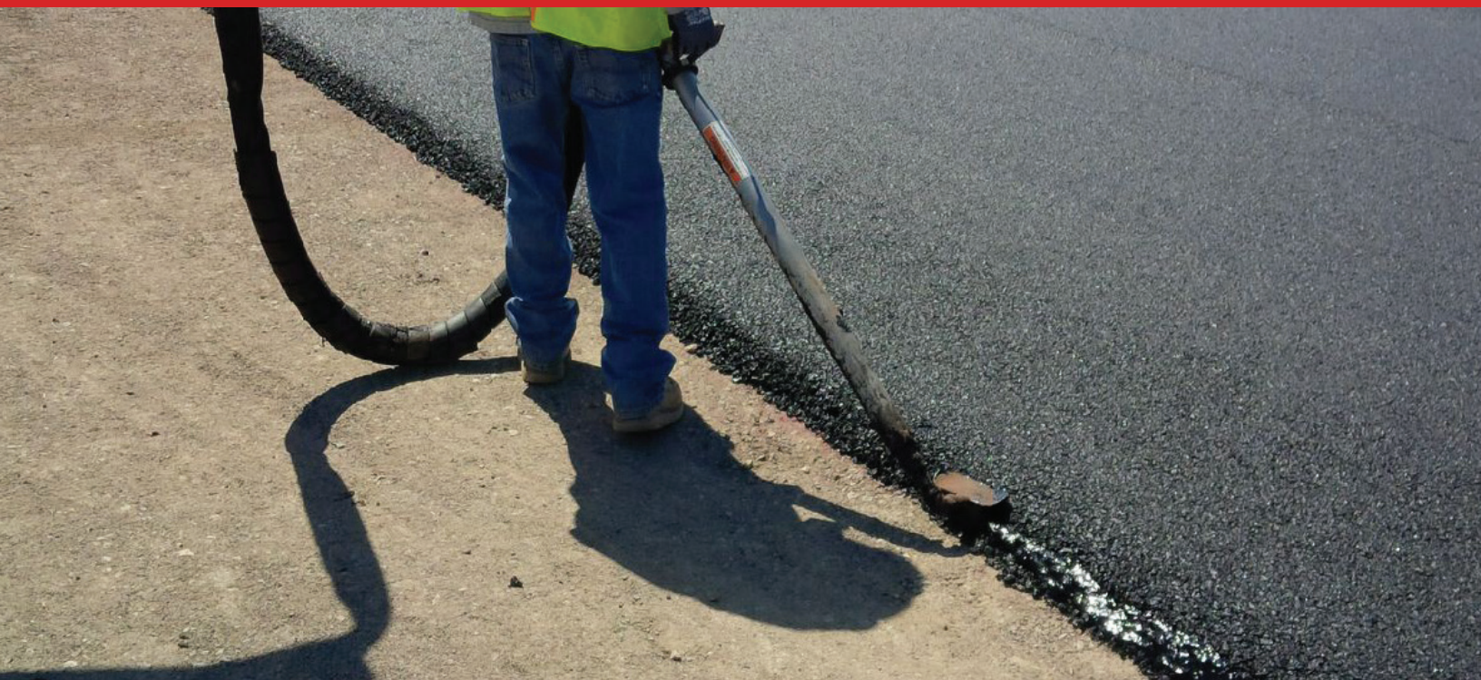
Application of cold joint adhesive
